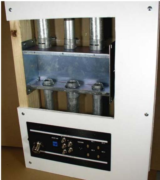
The **back-box** assembly will support all 1" or 1-1/4" conduit or a combination of both as shown in the picture to the above and to the left.
